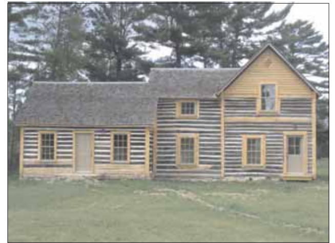
Dinesen house upon completion of restoration.
